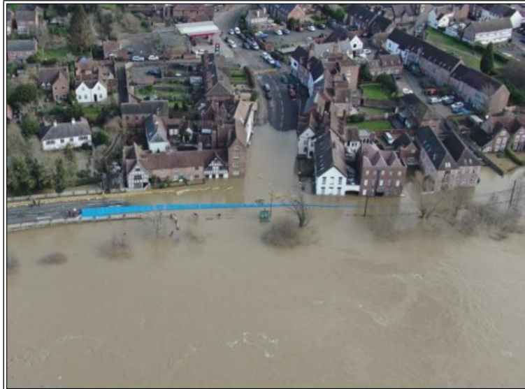
Figure 2: River levels outflanked the Beales Corner temporary barriers
