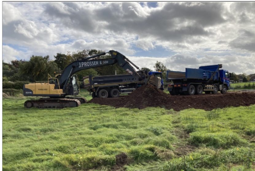
Figure 13: Soil being transported to Severn Stoke for use in the flood alleviation scheme. (Annex A, Table A2, item P7 refers.)
